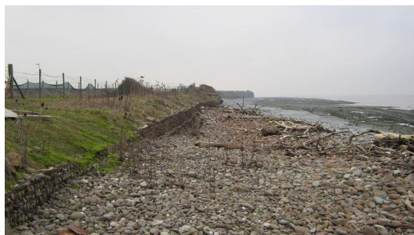
Storm damage to the coastline at Hinkley Point. Lots of debris washed up on the shore with more evidence of the gabions being damaged as well as new rock falls from the extremely fragile field edges all along that part of the coastal boundary.
